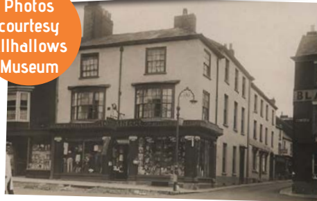
VIEW OF FORMER HOSKINS TAILORS
