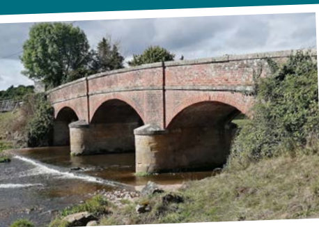
Weir at Gosford road bridge.
